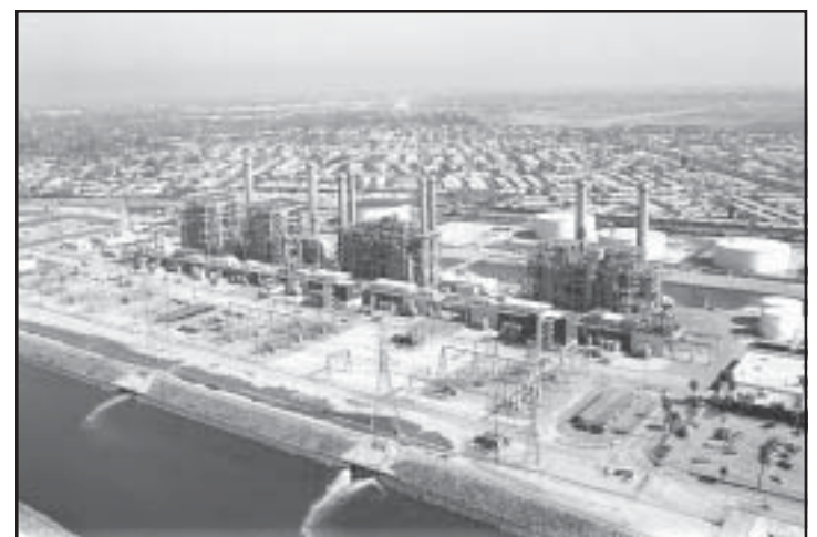
When completed the Haynes Power Plant in Long Beach will produce enough electricity to power 1.5 million homes.
